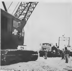
THE ENTIRE load is supported on forty-two wheels which keep the rig from sinking into the soft sand beach. Slowly, but surely, bottom photo, the rig moves toward the erection site. HENTER E carga ta wanta ariba cuarenta y dos wiel, cual ta tense e trailer pa e un ataca den e santu moti di lama. Poco-poco e trailer ta bai na su lugar.
